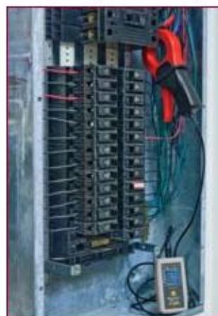
L101 recording branch circuit current.
